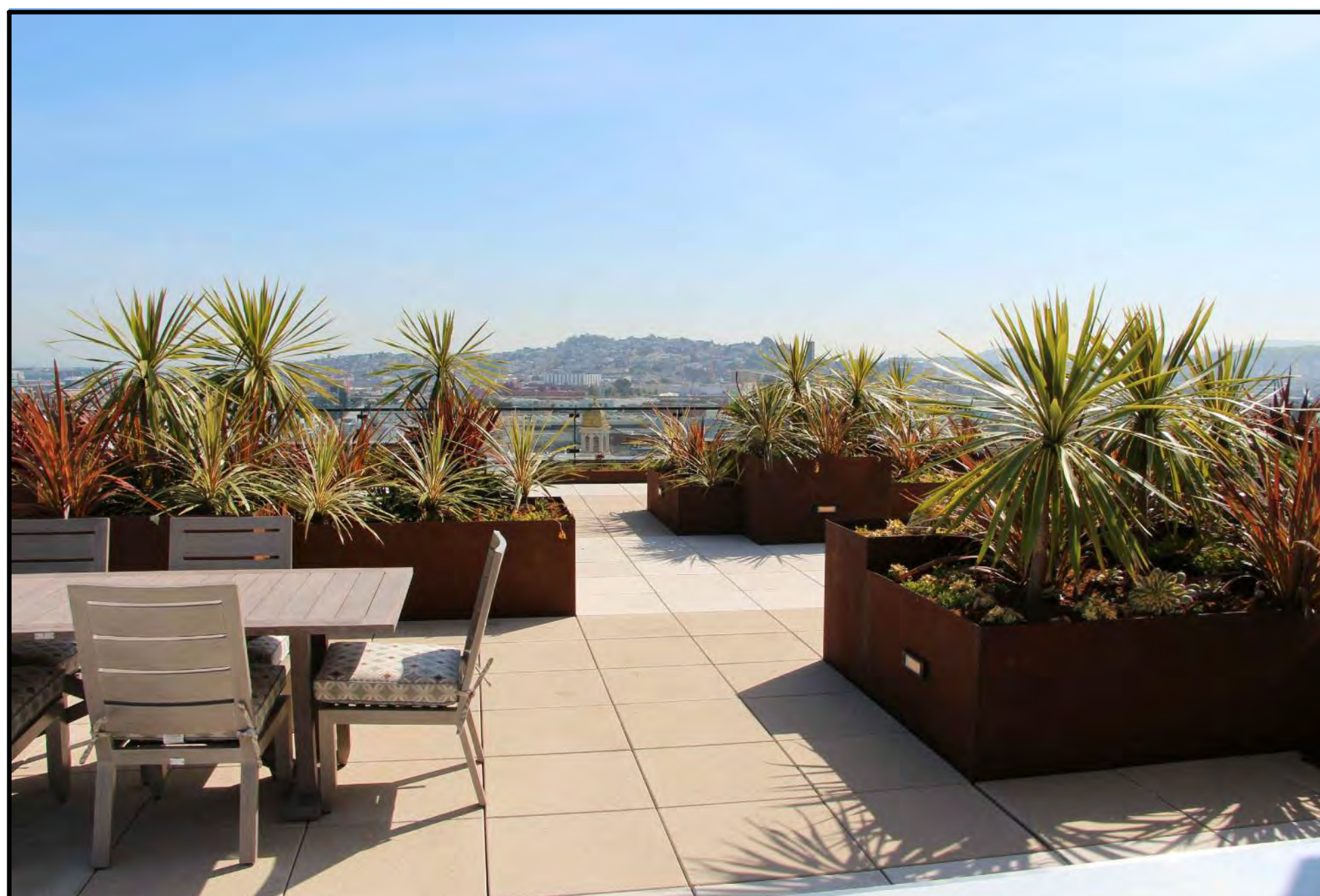
Steel Planters on Roof Terraces
