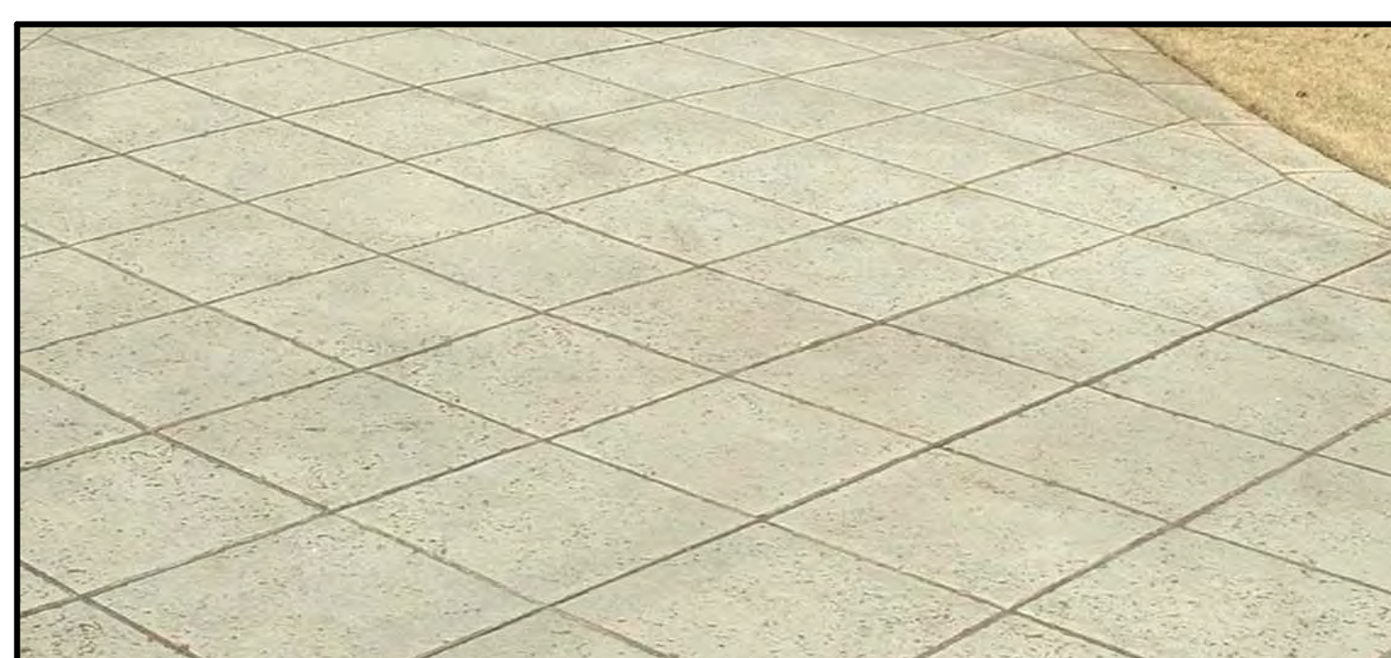
Vehicular Concrete Paving
