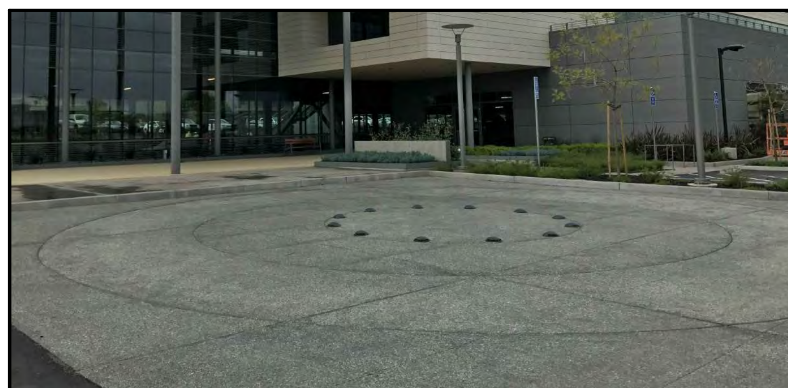
Drop off Concrete Paving
